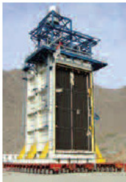
ME moving a 1200 tonne machine in UAE
